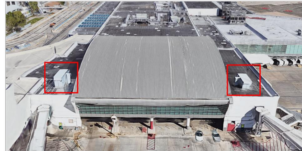
AHU 2-22/2-23 Replacement to XD or CHW connection to Terminal A Chiller Plant
