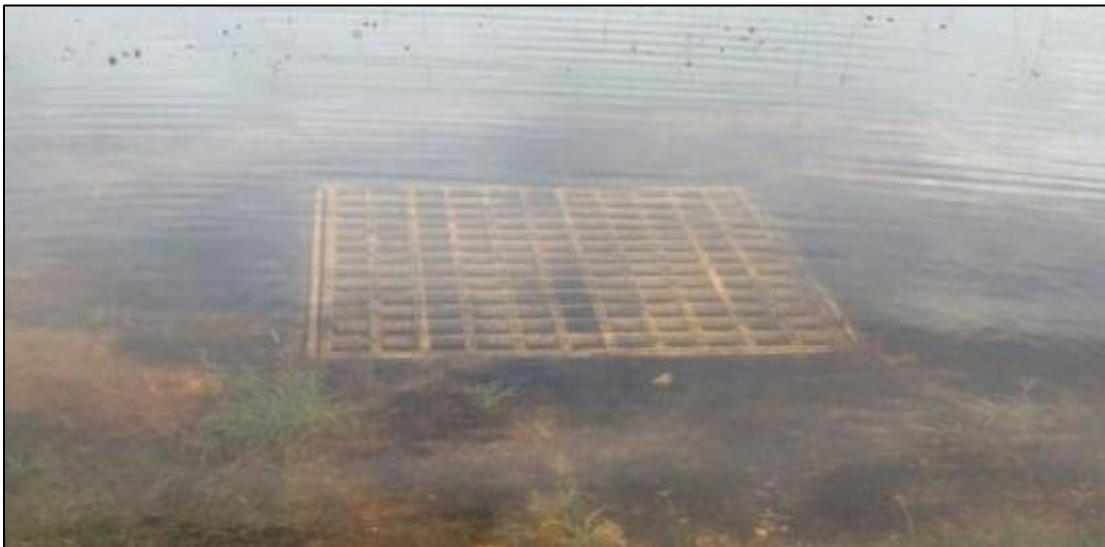
Photo 3 Ponding water above a stormwater inlet.
