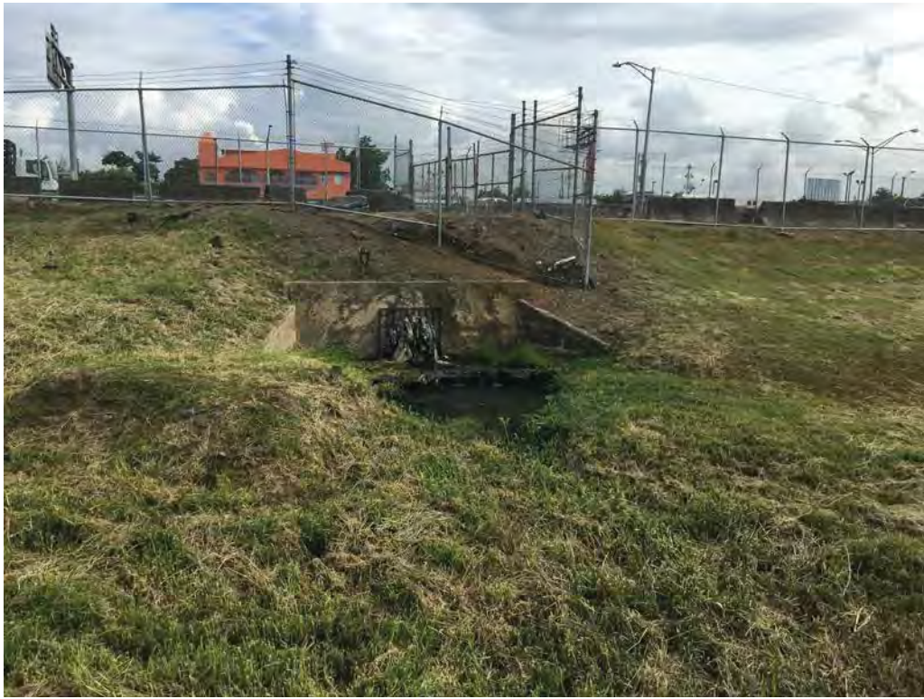
PHOTO 7 & 8: STORM WATER INLET AND DRAINAGE WETLAND AREA, SOUTH RUNWAY 10-28.
