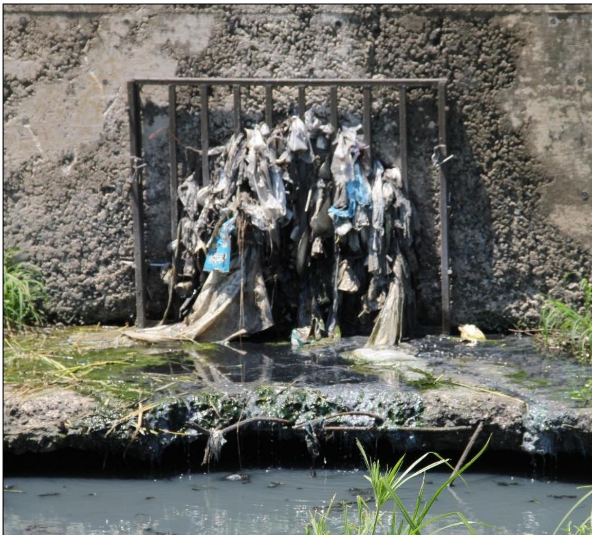
Photo 5 Clogged sanitary drain discharging into airport.
